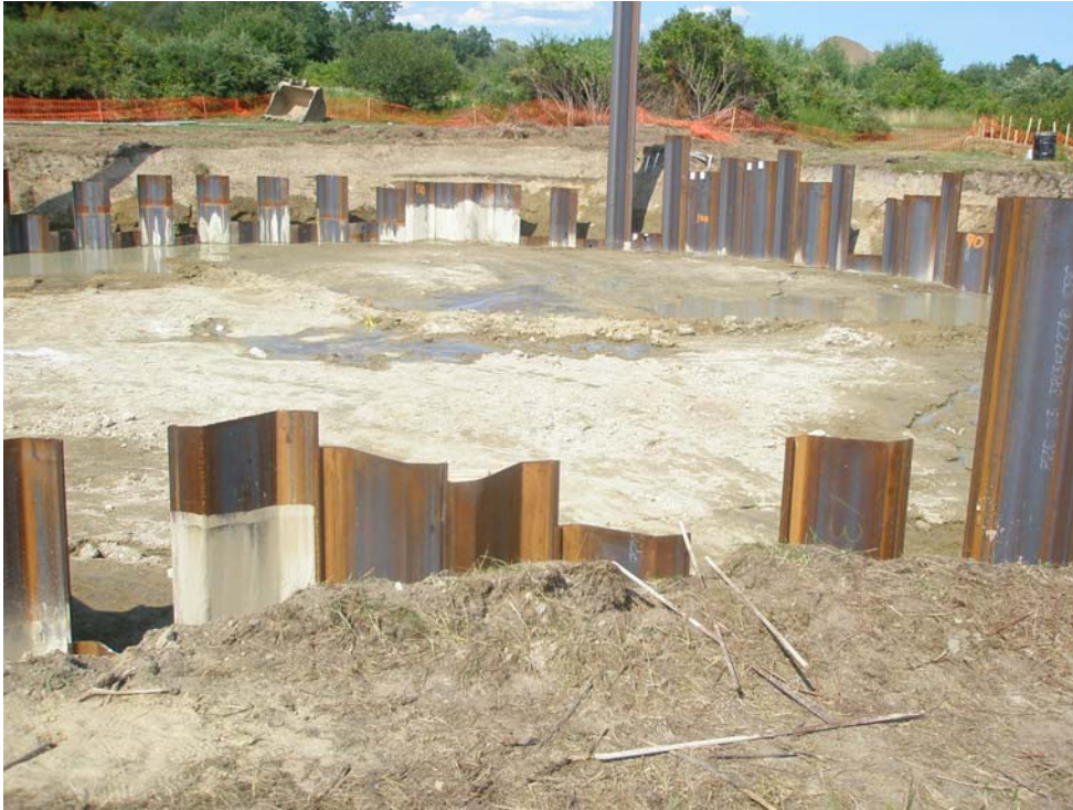
Photograph 1 – Adjustments Made to Sheet Pile
