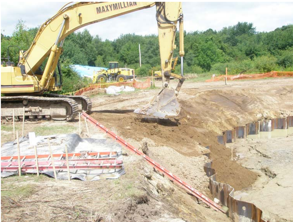
Photograph 2 – Creating Ramp for Access to Cofferdam Interior
