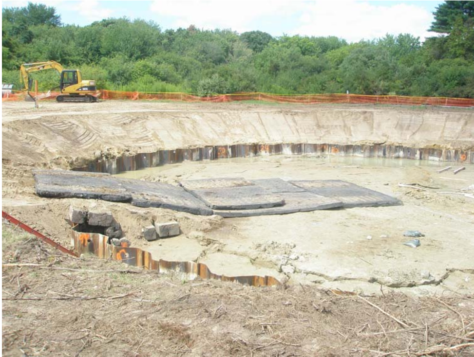
Photograph 3 – Completed Ramp with Tundra Mats
