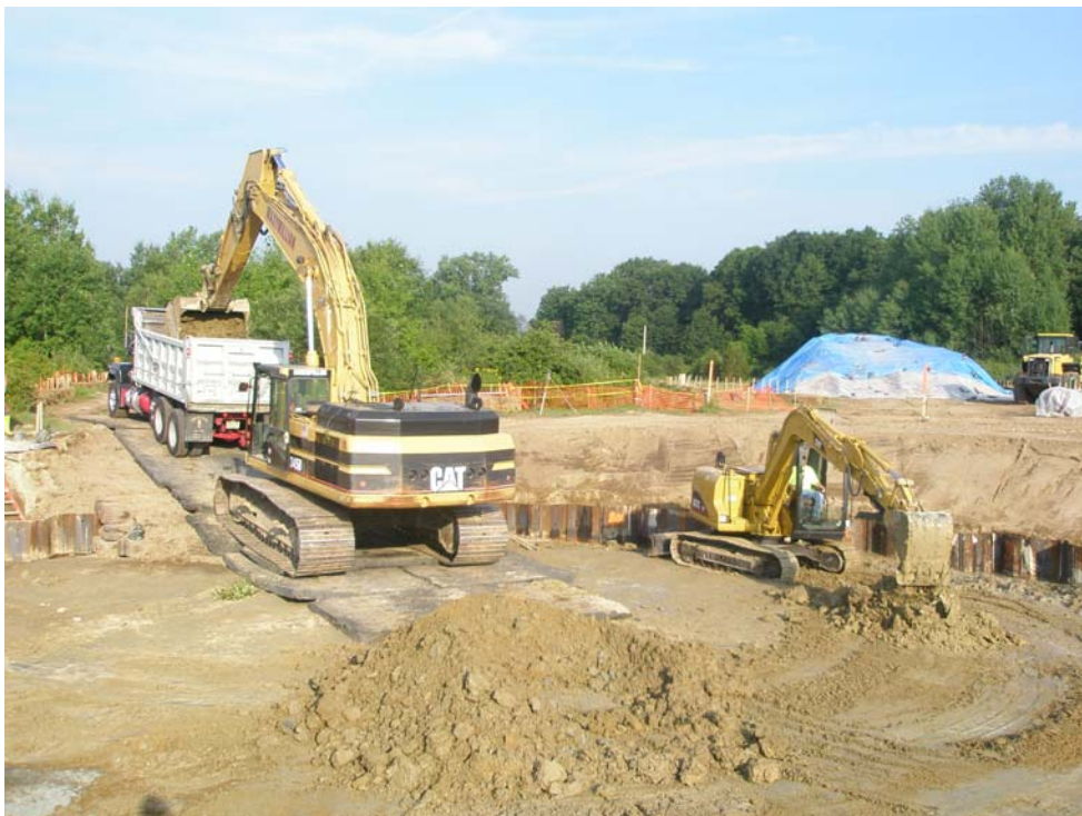
Photograph 4 – Beginning Excavation to 117' asl
