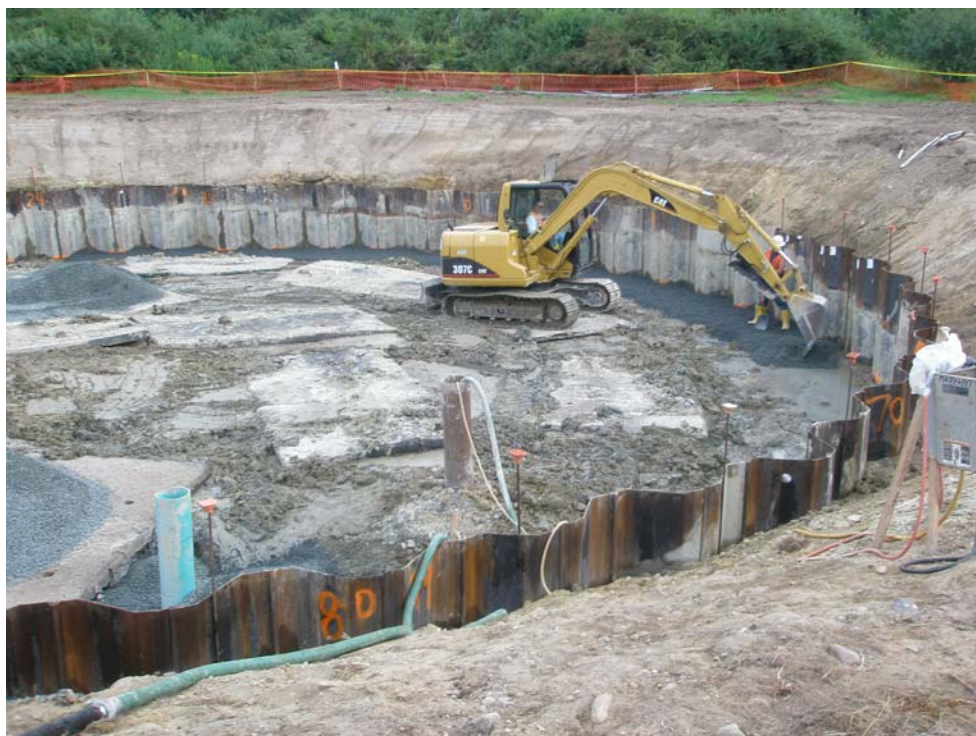
Photograph 6 – Crushed Stone Installed in Preparation for Concrete Wale
