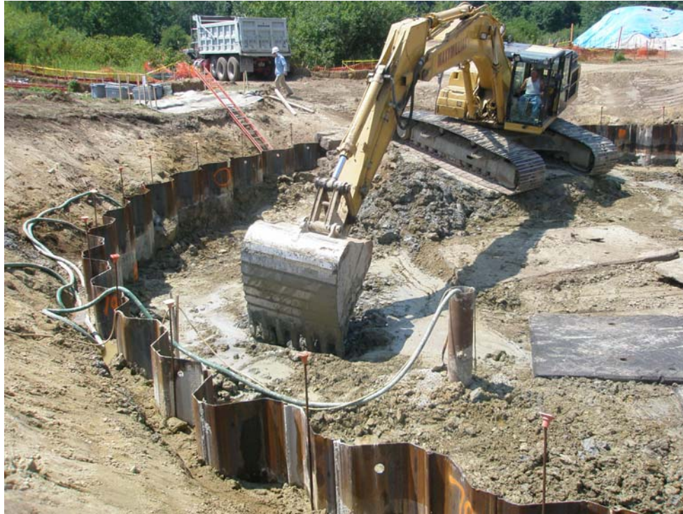
Photograph 5 – Continued Excavation and Dewatering
